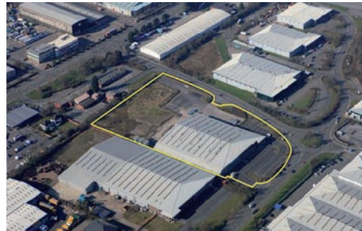
Parc Nantgarw, Treforest, South Wales Leasehold acquisition of 57,000 sq ft factory for conversion to bus depot on behalf of Veolia Transport.
