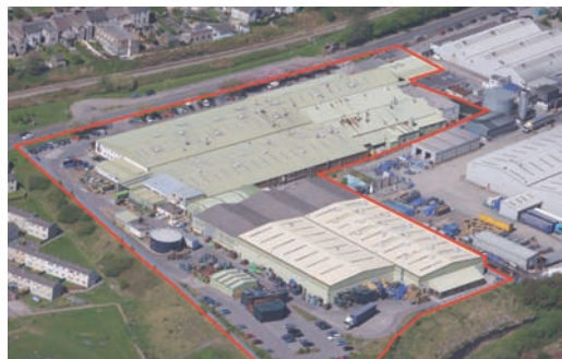
Ewenny Industrial Estate, Maesteg, South Wales Freehold disposal of 163,000 sq ft factory on behalf of Cooper Standard Automotive.
