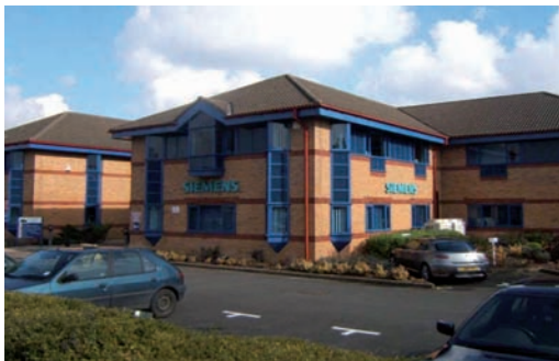
Highlands Court, Solihull Leasehold disposal of 2,151 sq ft office on behalf of Siemens Real Estate.
